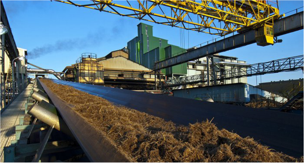
In Swaziland, bi-products of refining sugar are used to generate electricity
