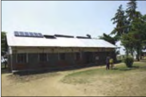
Solar panels provide electricity to Kalungi Hospital.
